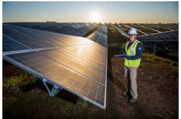
Bill Gatherwright checks one of the 32,000 panels in Cooperative Solar Farm One, which was built last year by Fleming-Mason Energy and Kentucky's Touchstone Energy Cooperatives. Photo: Tim Webb
